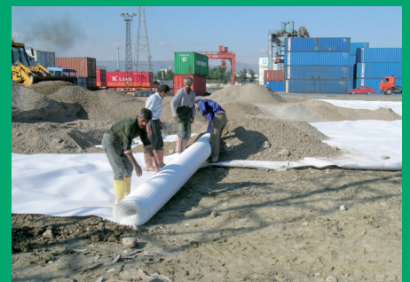
Figure 5 Unrolling and overlapping of Combigrig® over the soft subgrade
