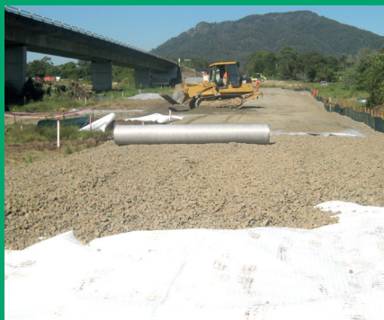
Figure 4 Combigrig® unrolled and covered with topsoil
