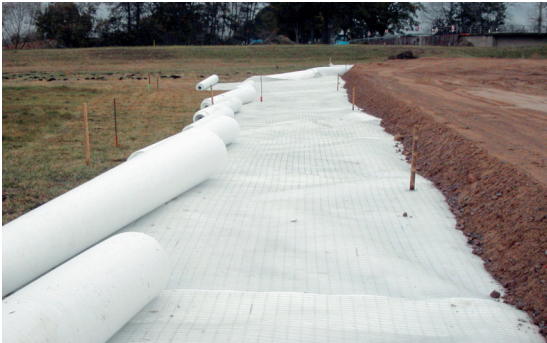
Installed Combigrid® with overlaps
