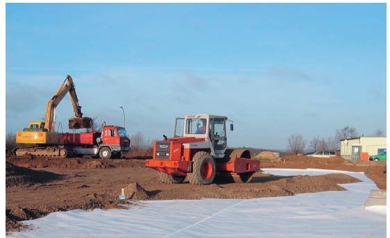
Soil compaction over Combigrid®
