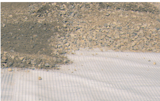
Aggregate interlocking
